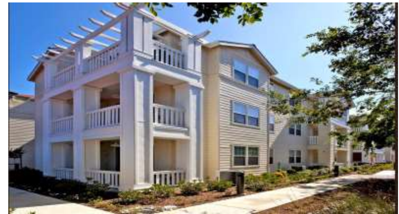
Casa del Maestro is a 70-unit residential development providing apartments affordable to teachers of Santa Clara unified school district.
