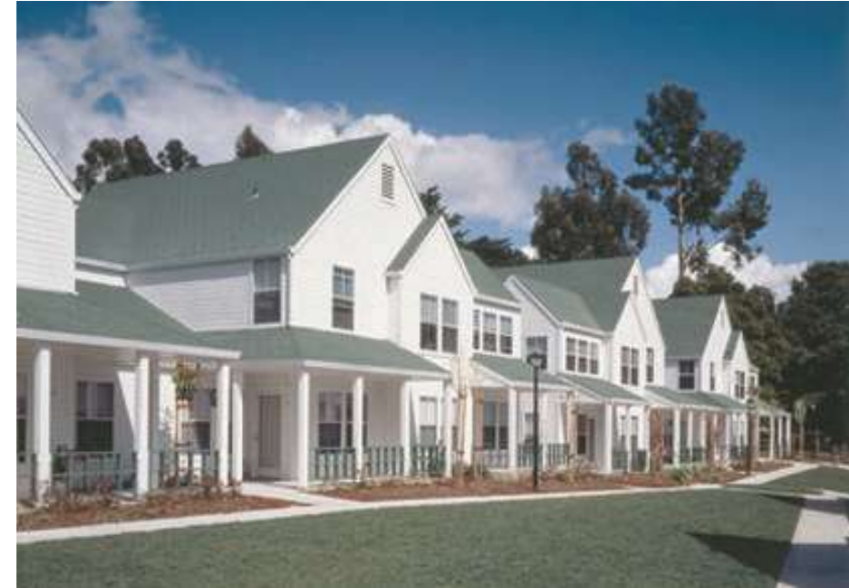
The Farm, MidPen Housing, County of Santa Cruz Redevelopment Agency.
